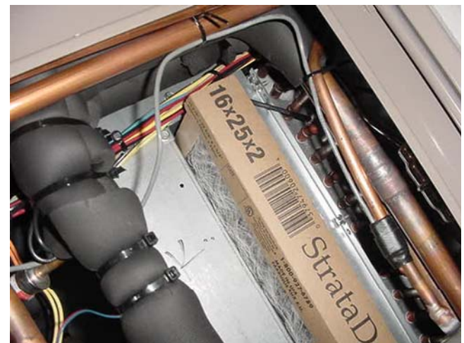
FIGURE 2 - SENSOR LOCATION FILTER SECTION
