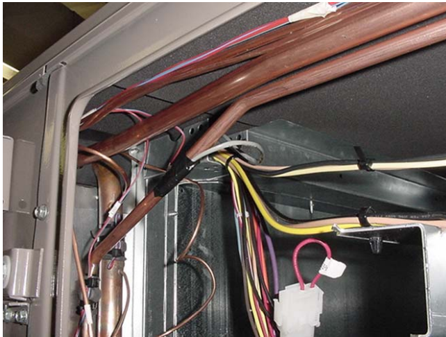
FIGURE 3 - SENSOR LOCATION BLOWER SECTION
