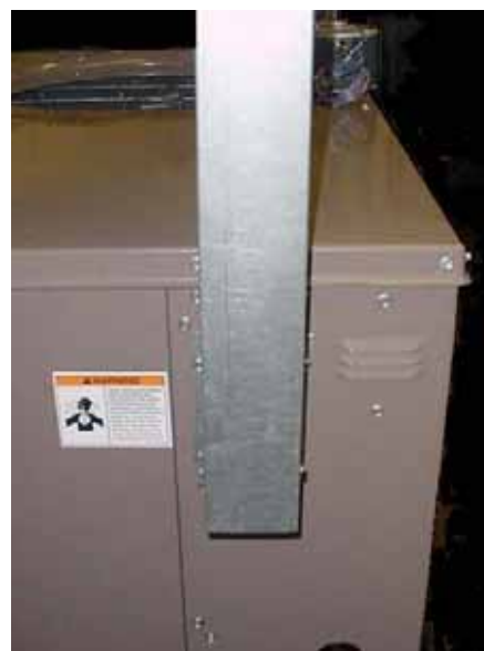
FIGURE 3 - INSTALL FLUE EXTENSION
