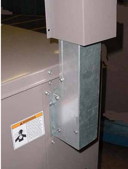
FIGURE 4 - SLIDE FLUE COVER OVER EXTENSION
