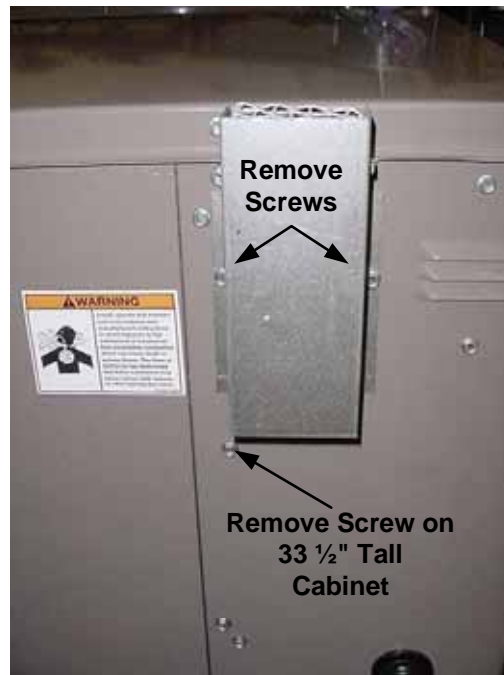
FIGURE 2 - ORIGINAL FLUE REMOVAL
