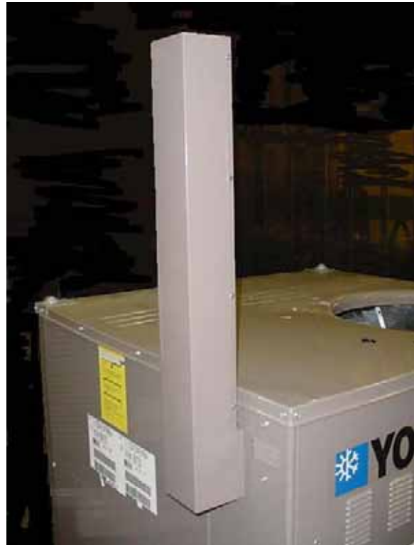
FIGURE 6 - FLUE COVER INSTALLED
