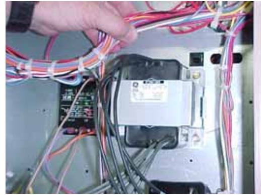
FIGURE 14 - Transformer
