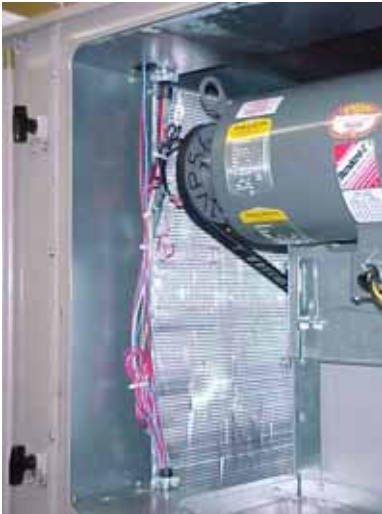
FIGURE 8 - Blower Section Wiring
