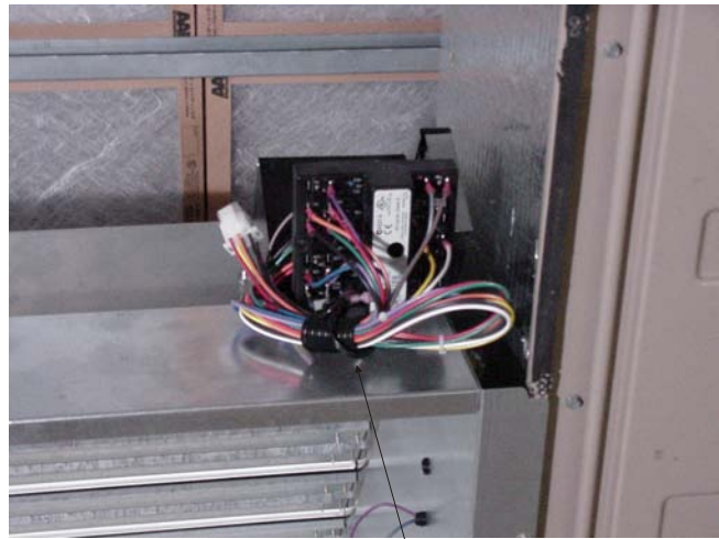
DISCHARGE AIR SENSOR
